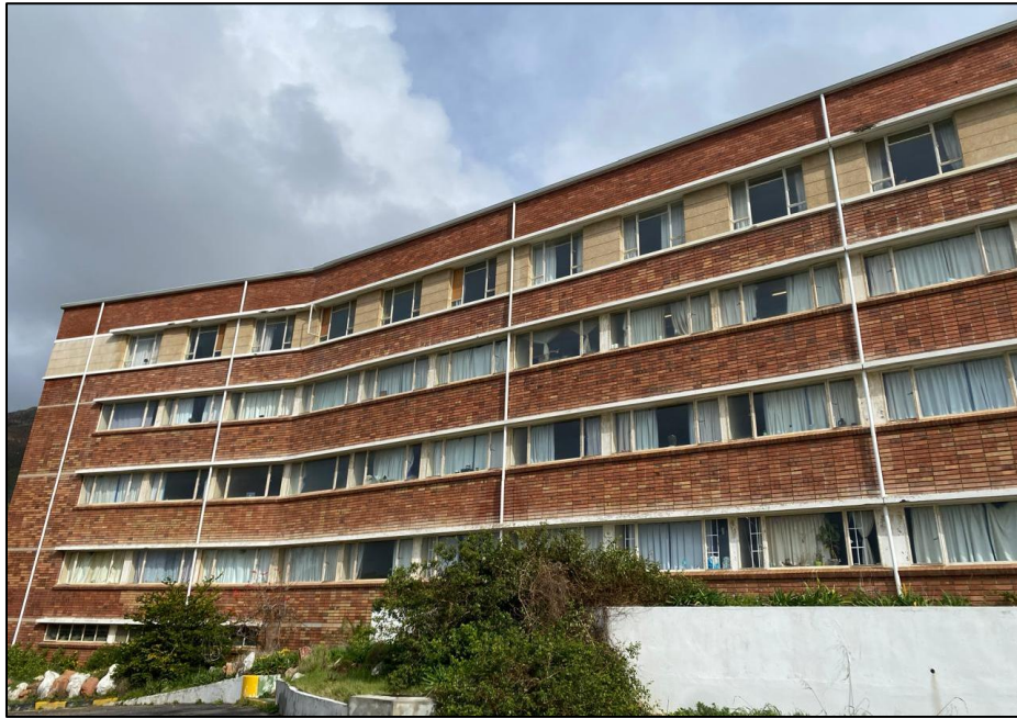
Figure 7. Broken windows at Job Maseko Wardroom have been replaced or boarded up.
