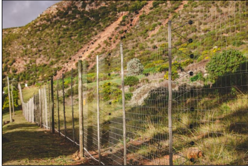
Figure 9. A section of the Zwaanswyk baboon-proof electric fence - Photo Charl Steenkamp.
